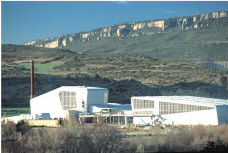
**Photo 1: View of the Sangüesa Power Plant with straw barn on the right, and boiler building on the left**
