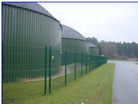
Figuur: vergister/ontzweveling/gasbuffer
