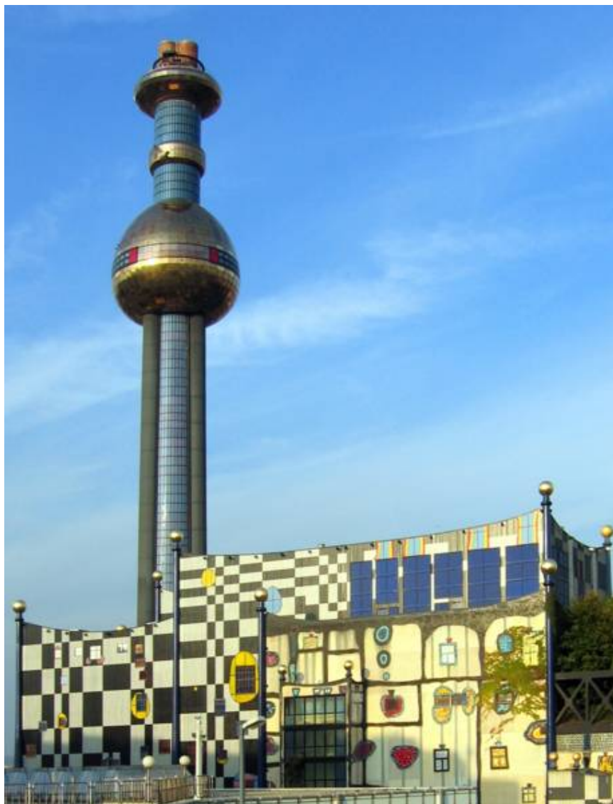
Waste incinerator that provides district heating in Vienna.
