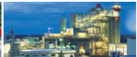
Uruguaiana, Brazil: 600 MW combined cycle power plant with two W501F (new: SGT6-5000F) gas turbines in 2x1 multi-shaft configuration
