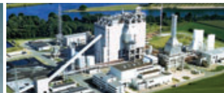
Buggenum, Netherlands: 290 MW IGCC power plant with one V94.2 (new: SGT5-2000E) gas turbine for both syngas and natural gas application
