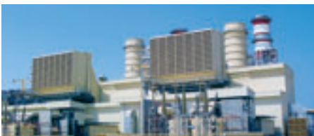
Shuweihat S1, United Arab Emirates: 1,500 MW combined cycle power plant with desalination using five V94.3A (new: SGT5-4000F) gas turbines in a multi-shaft configuration
