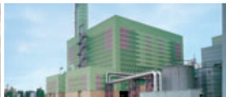
Mainz-Wiesbaden, Germany: 400 MW combined cycle cogeneration power plant using one V94.3A (new: SGT5-4000F) gas turbine
