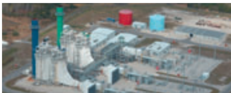
Payne Creek, Florida, USA: 515 MW combined cycle power plant with two W501F (new: SGT6-5000F) gas turbines in 2x1 multi-shaft configuration
