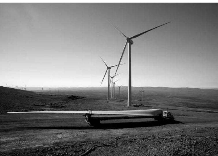
Wild Horse wind farm, Ellensburg, Washington, USA © Renewable Energy Systems Group
