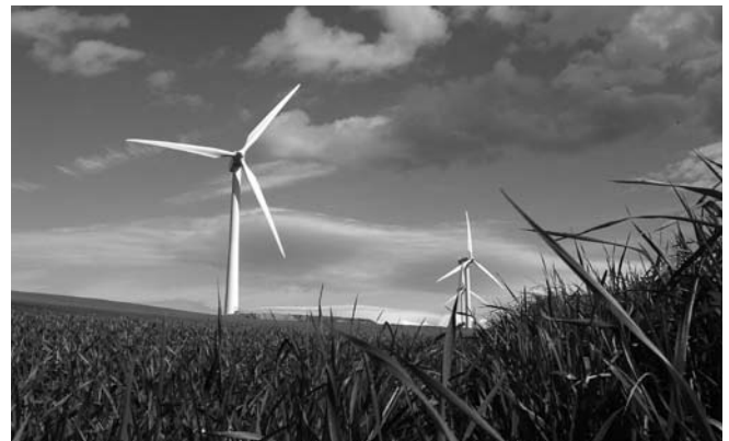
Whitelee wind farm © Scottish Power
