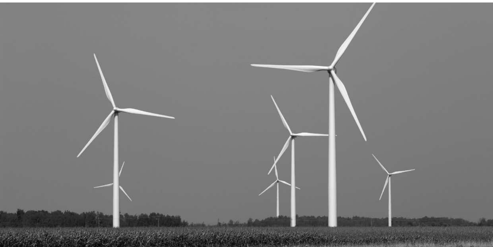
Melanchton wind farm in Shelburne, Ontario © CanWEA
