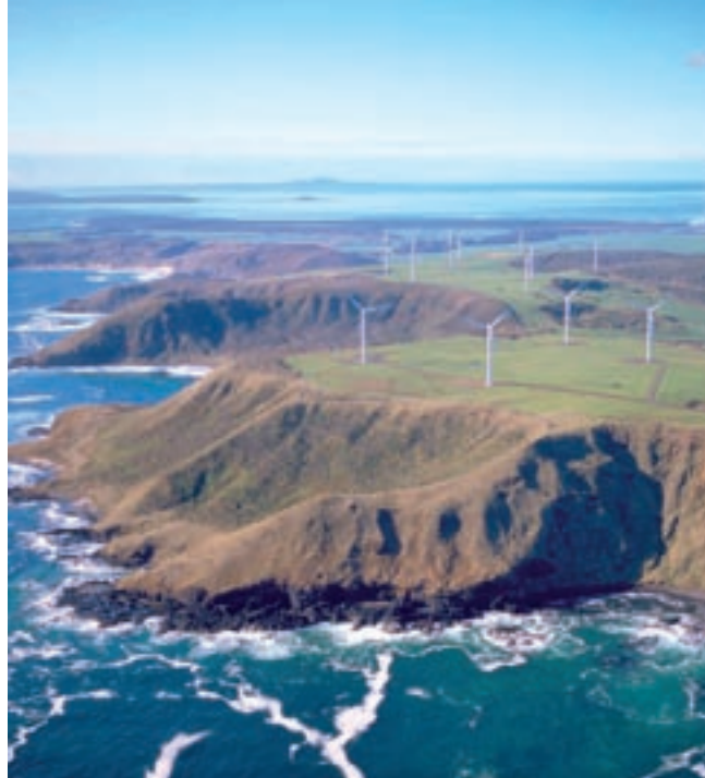
Woolnorth wind farm (Photo: Roaring 40s)
