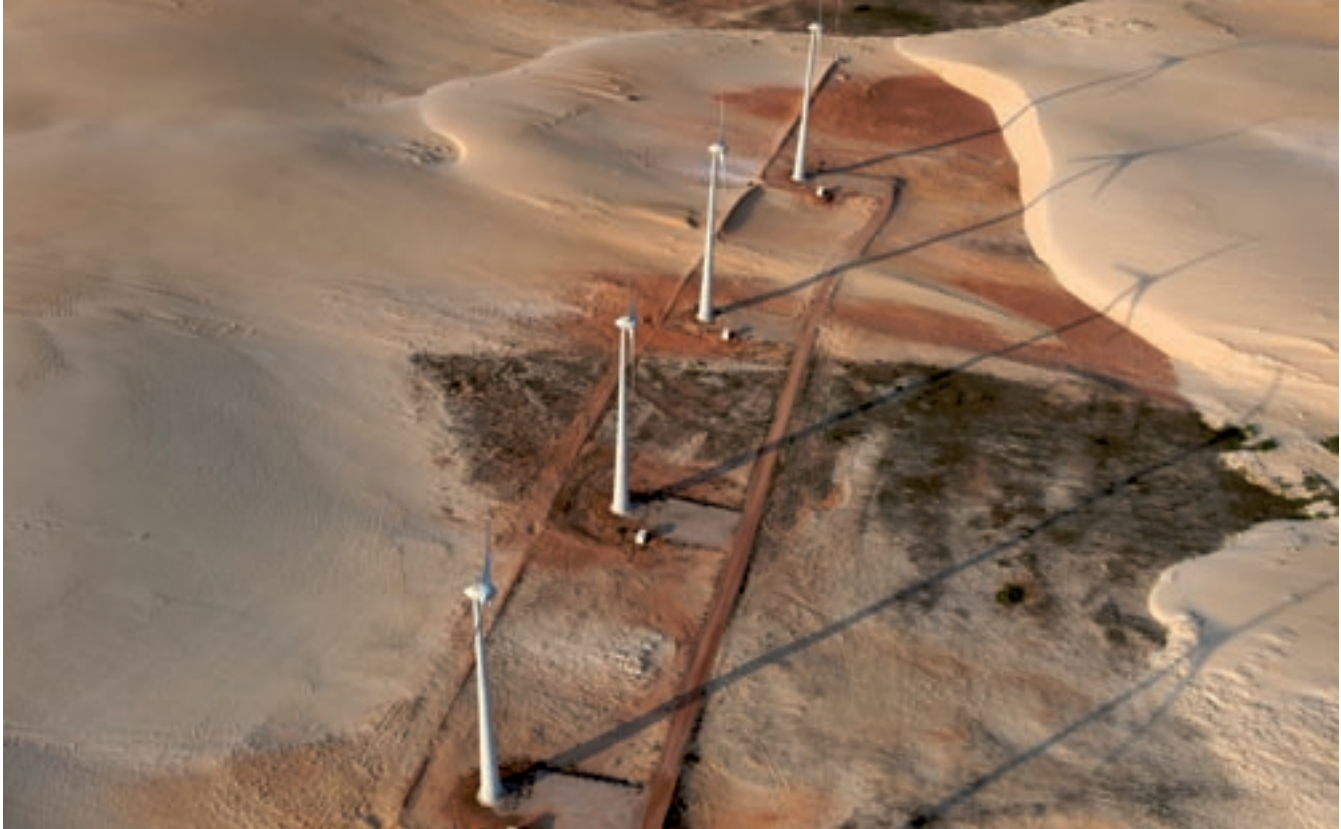
Brazil, Rio do Fogo wind farm (Photo: Wind Power Works)
