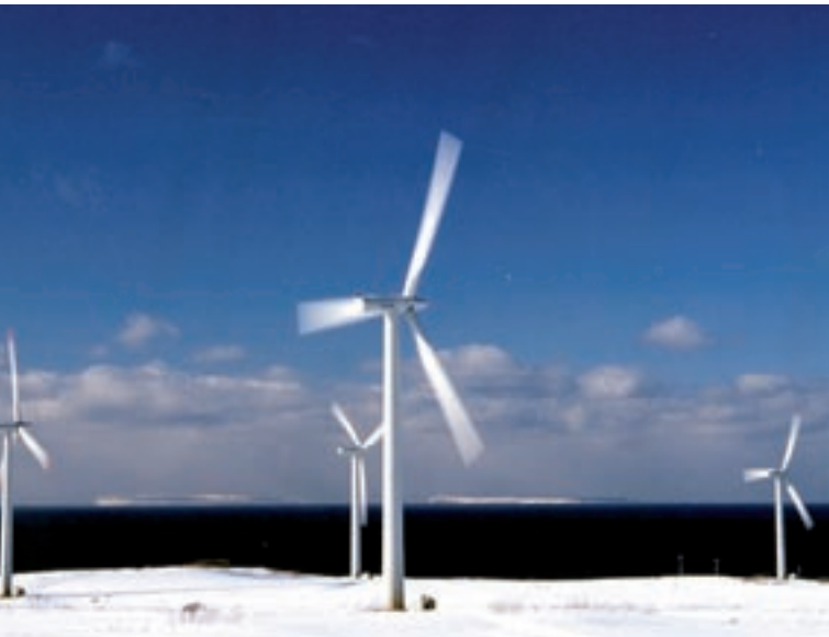
Tomamae wind farm (Photo: Japanese Wind Energy Association)
