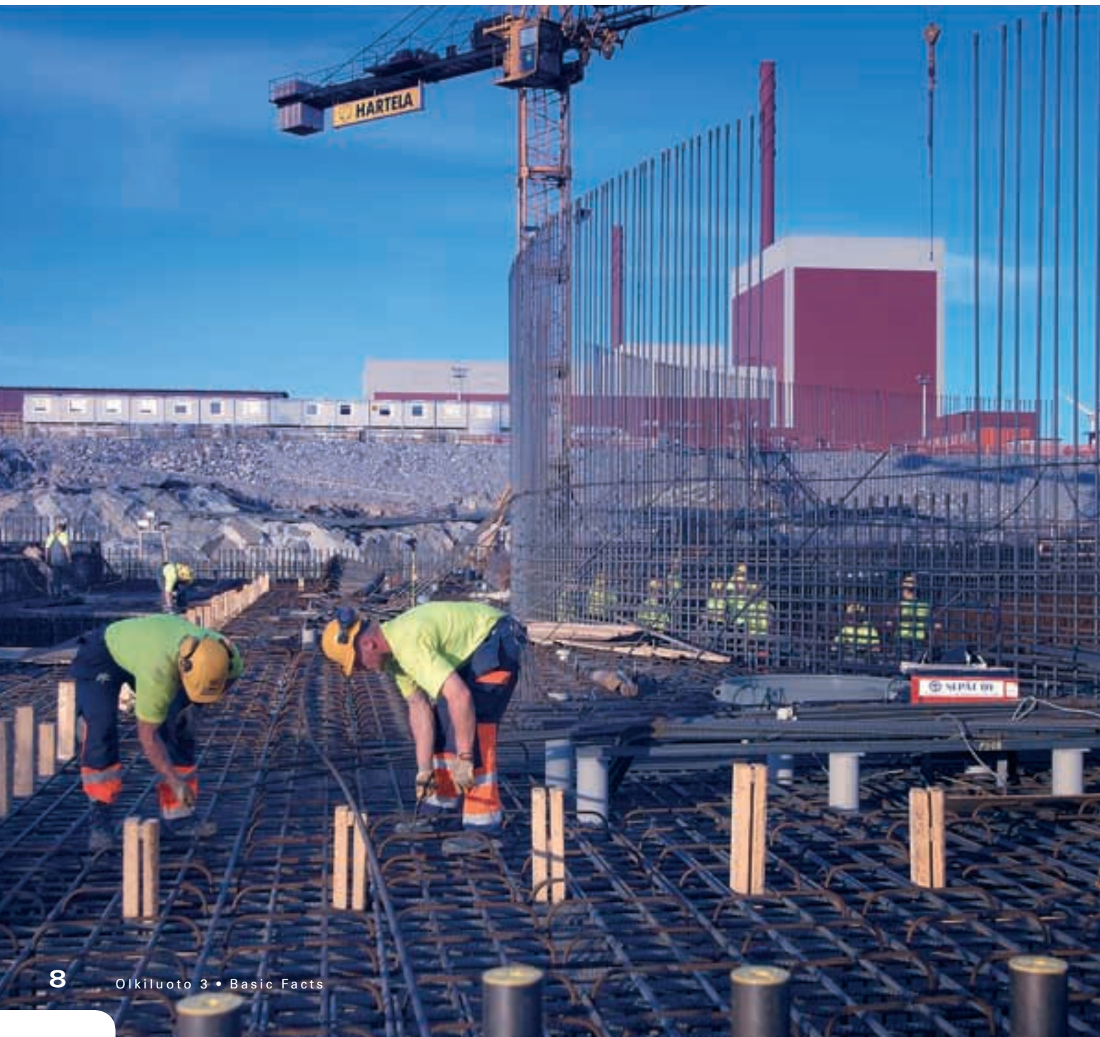
Reinforcement steel installed for the base slab in July 2005.
