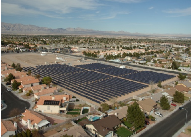
Figure 4 - SunPower's T0 Tracker
