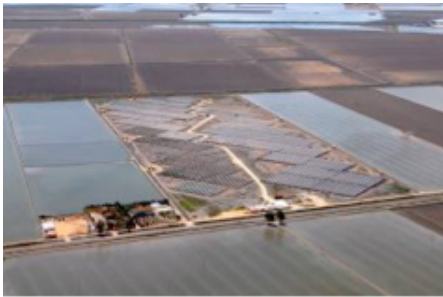
Isla Mayor Spain, 8.4 MW SunPower T0 Tracker
