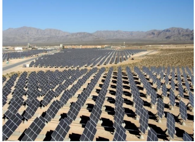
Figure 5 - SunPower's T20 Tracker
