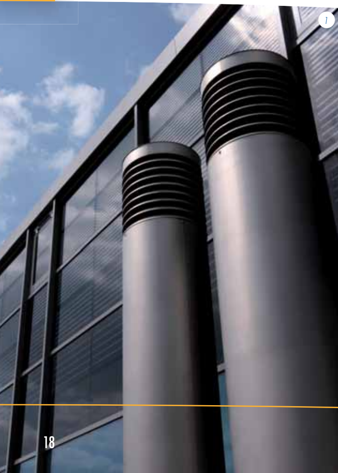
1. Semitransparent CIGS façade with varying transparency in insulated glass panels and with invisible junction boxes the sports arena of Anne-Sophie-School (Künzelsau, Germany) ©WURTH SOLAR
