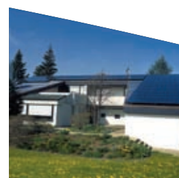
Roof mounted PV system with copper-indium-diselenide modules Source: Würth Solar
