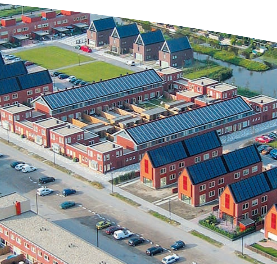
Roof mounted PV system with copper-indium-diselenide modules Source: Würth Solar
